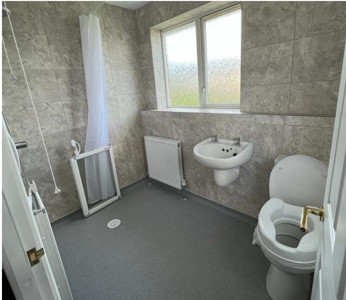
Level Access Shower Room funded through HEART with accessible wash basin and WC.
