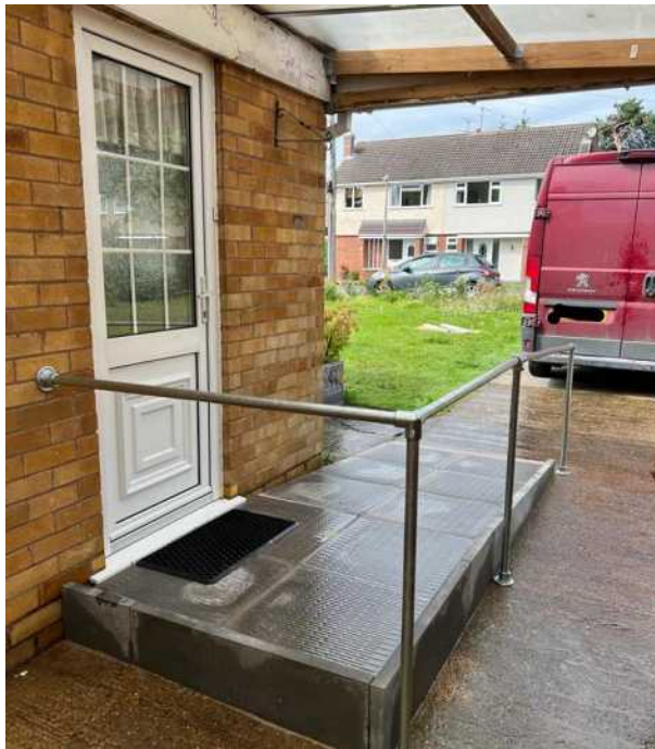
HEART funded access ramp and low threshold door.
