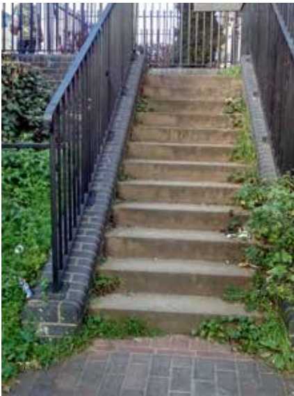
Stepped access Leamington Spa (WDC)
