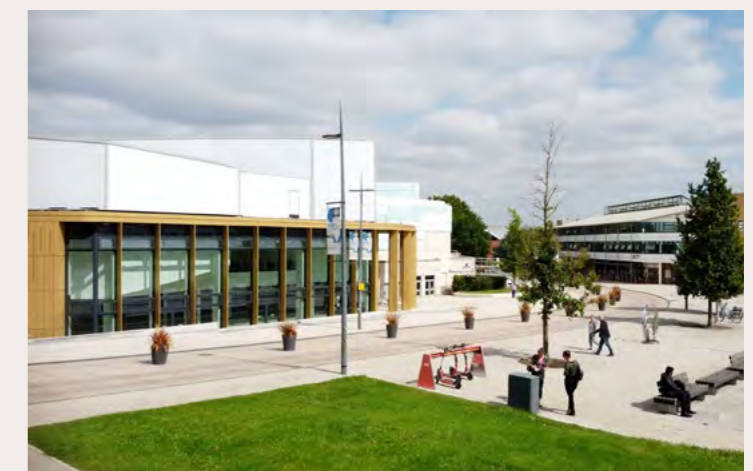
PHOTO 09: Warwick Arts Centre extension
