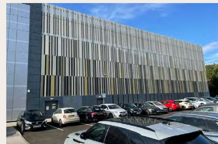
PHOTO 08: New multi-storey car park at Lynchgate
