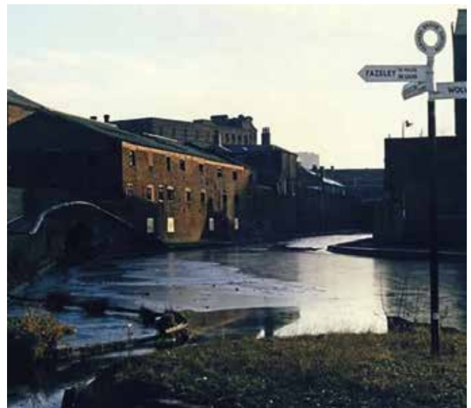
Before Work Started in 1990s at Brindley Place (Birmingham Express & Star)
