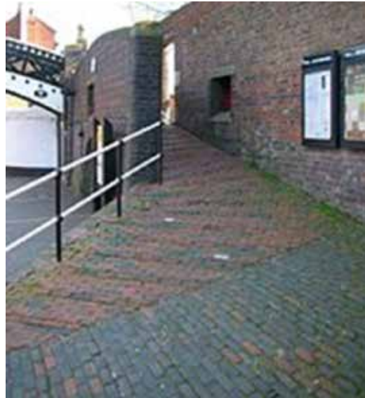
Improved access at Gas Street Basin (Oosoom)
