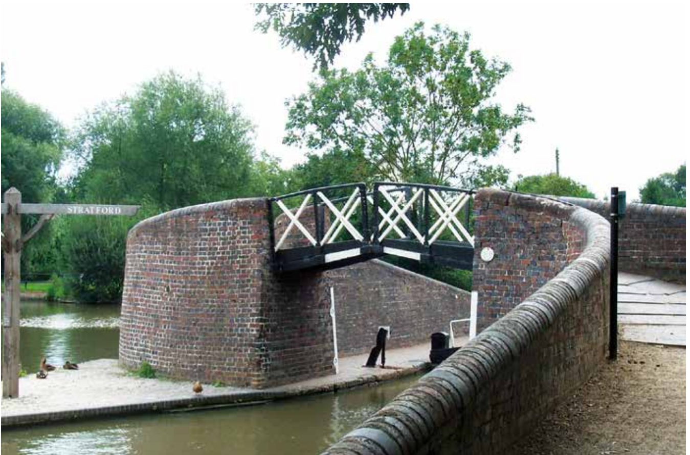
Split Bridge 2m North of Lock 21 (WDC)
