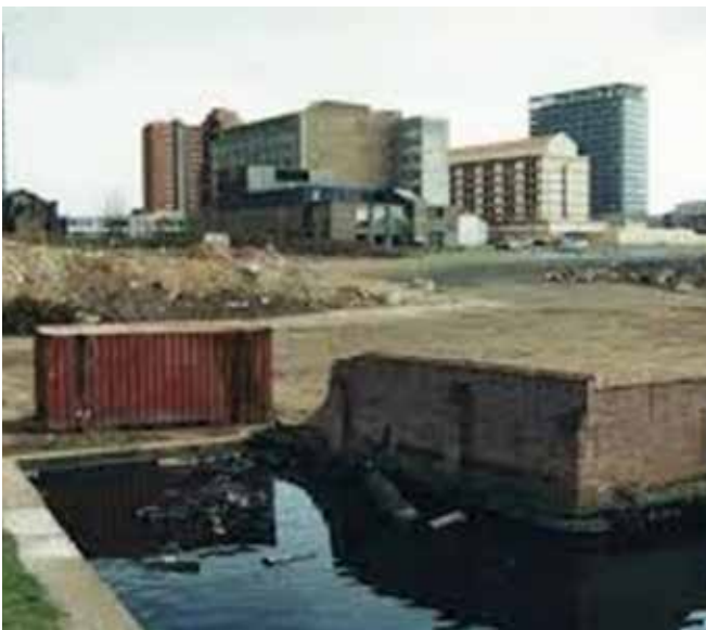
Brindley Place before work was carried out (Urban Buildings)
