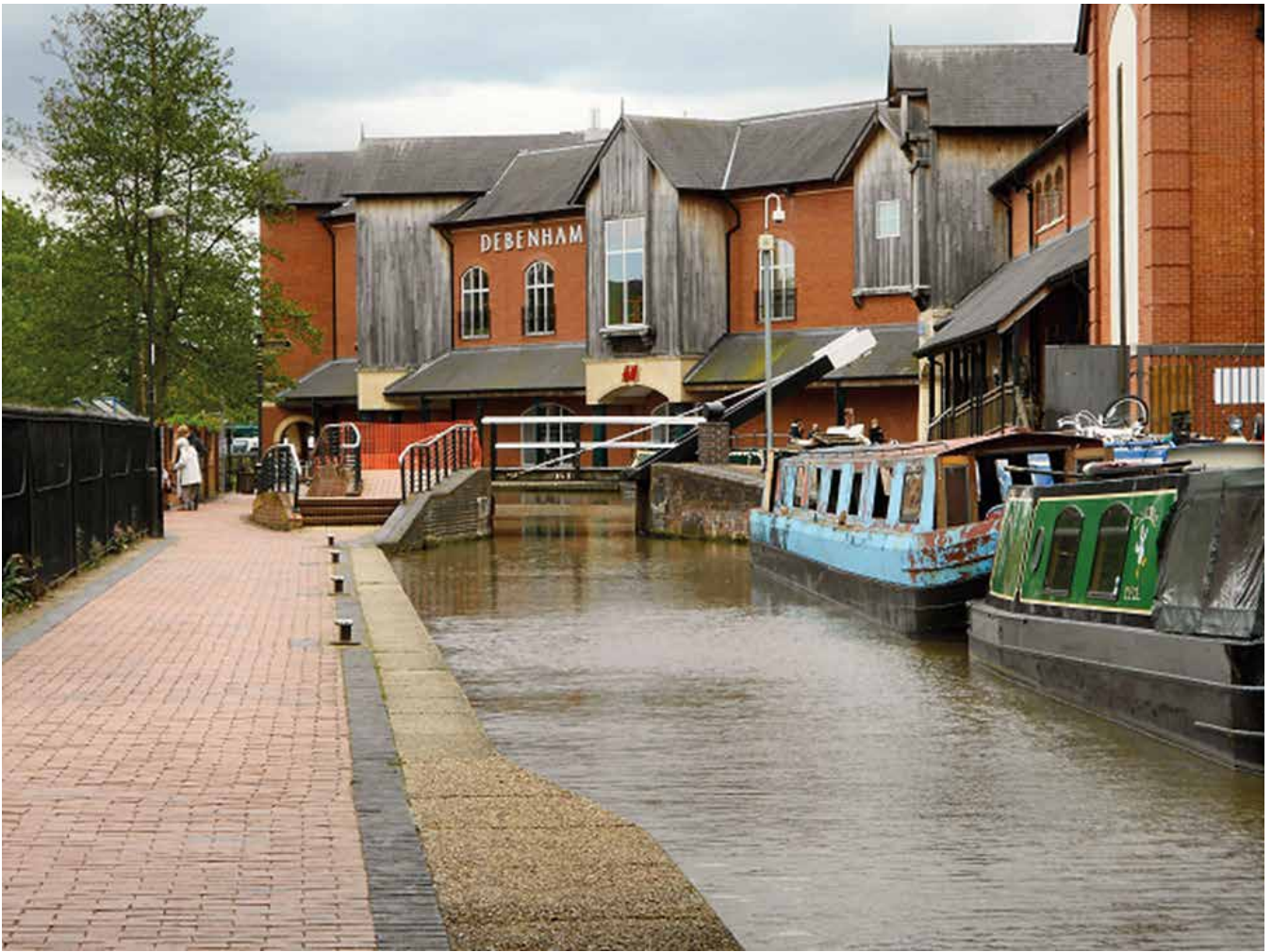
Banbury's Castle Quay – note the architectural features reflecting previous buildings/uses (Geograph)
