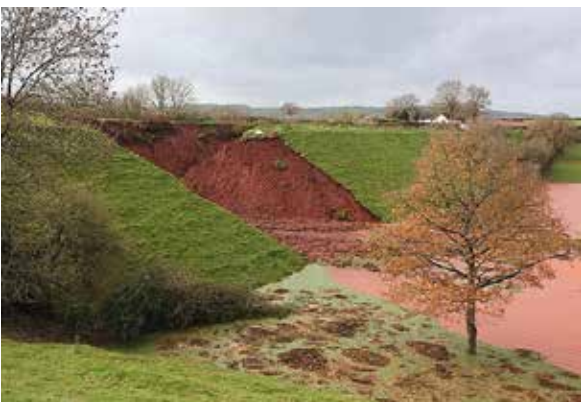
Great Western Canal, Devon, broke its banks in November 2012 (The Sun)
