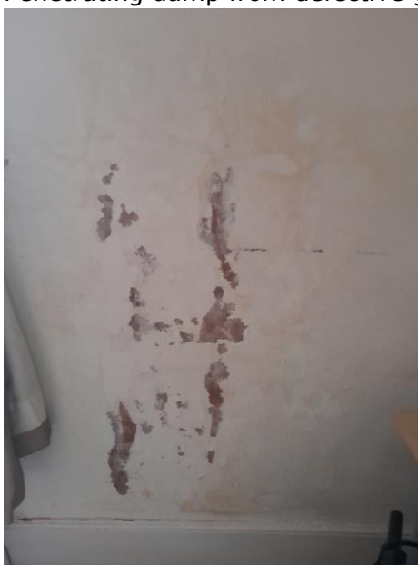
Penetrating damp from defective guttering
