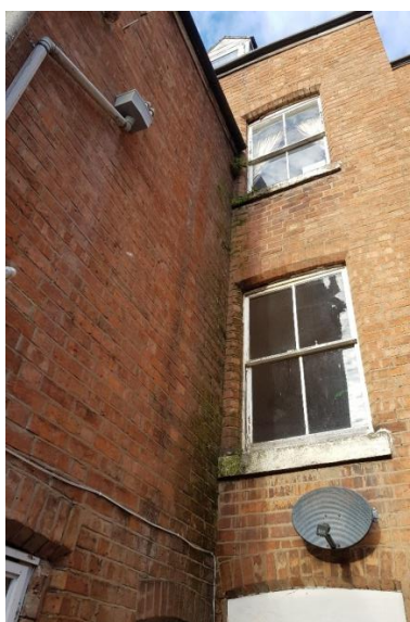
Penetrating damp from defective guttering
