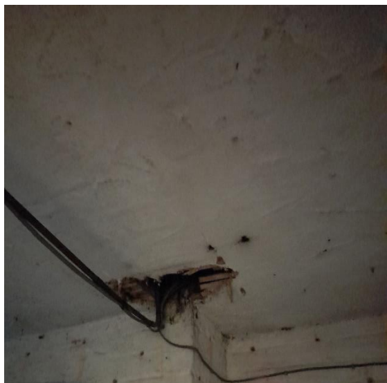
Service penetration hole in lath & plaster ceiling
