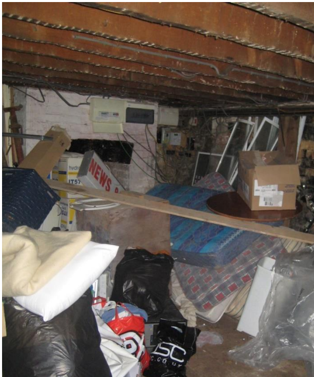
Accumulation of combustible material in cellar
