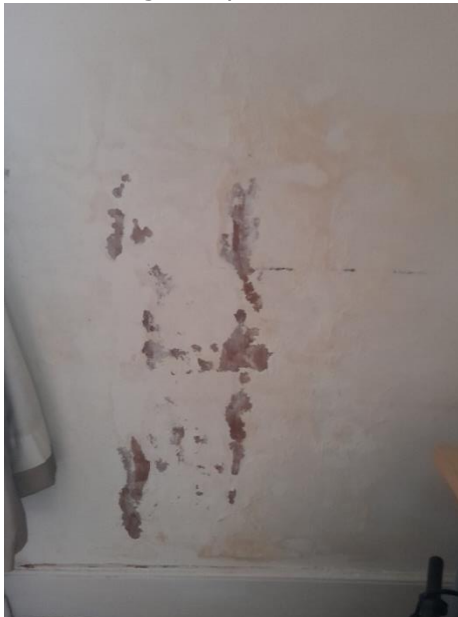
Penetrating damp from defective guttering
