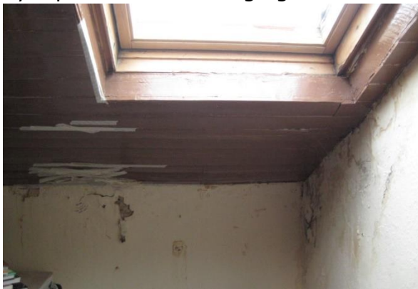
Leaking roof around roof-light in bedroom
