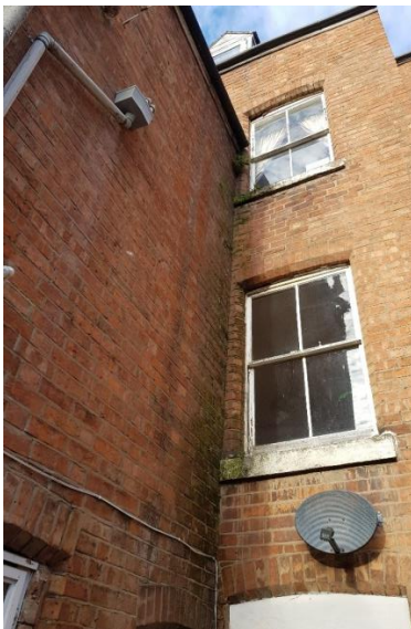
Penetrating damp from defective guttering
