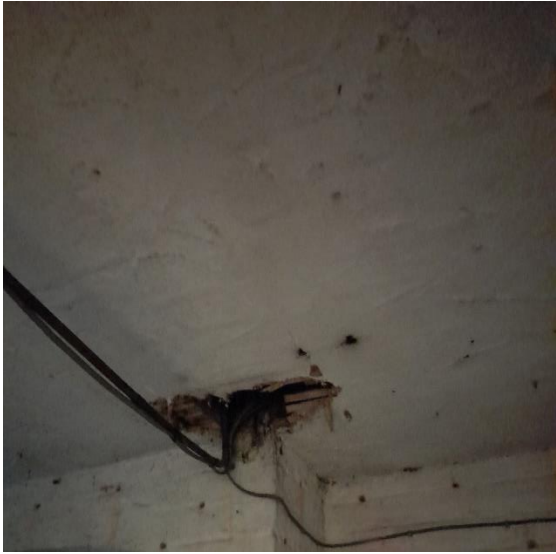
Service penetration hole in lath & plaster ceiling
