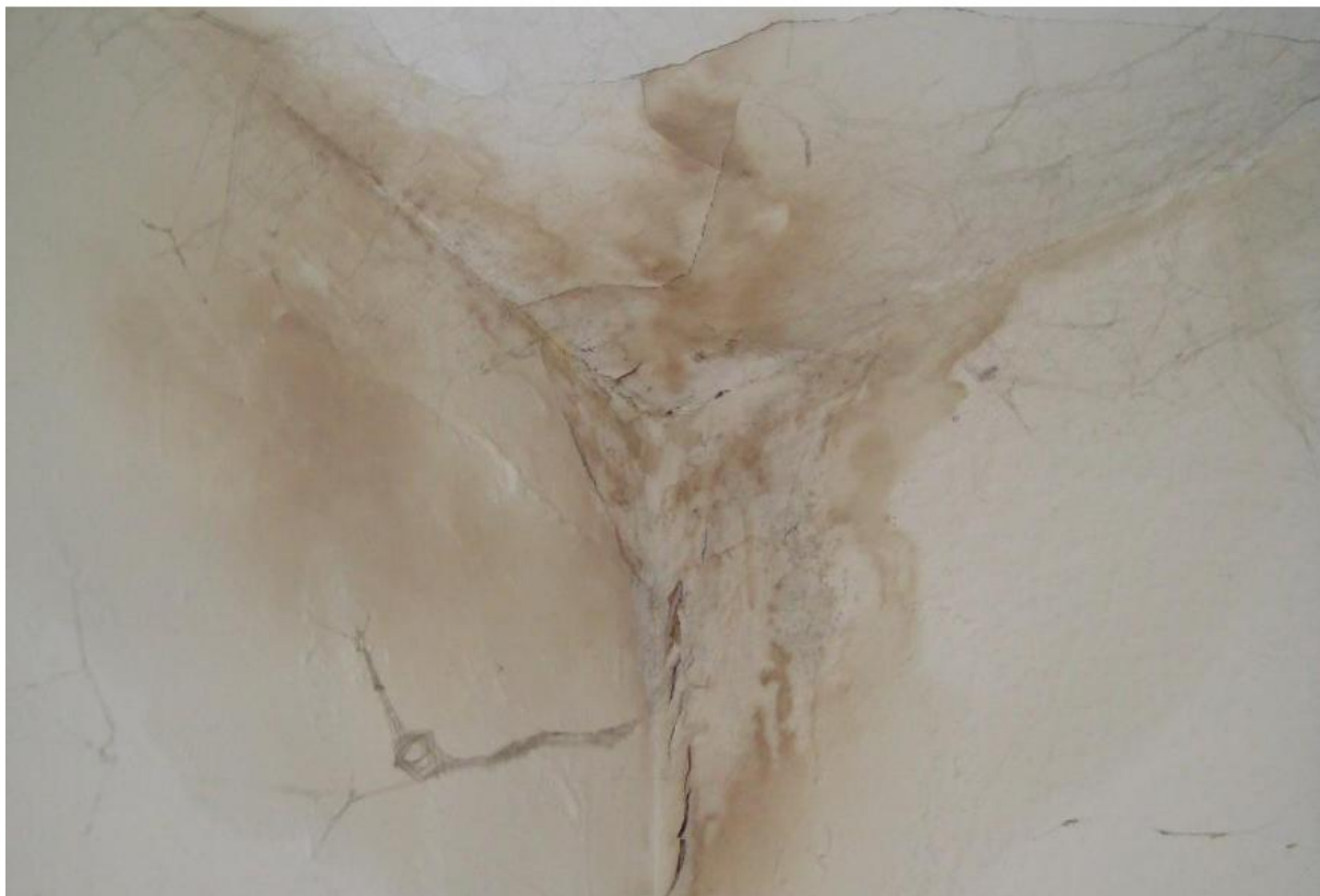
Damp penetration from leaking shower
