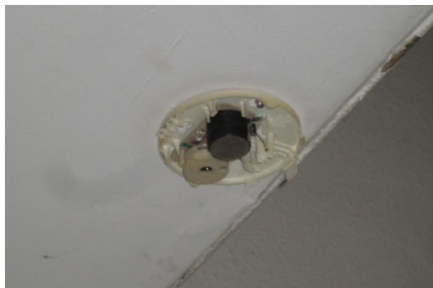
Defective smoke detector
