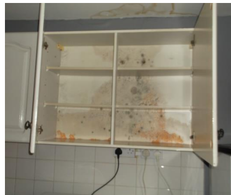
Penetrating damp to kitchen wall and ceiling
