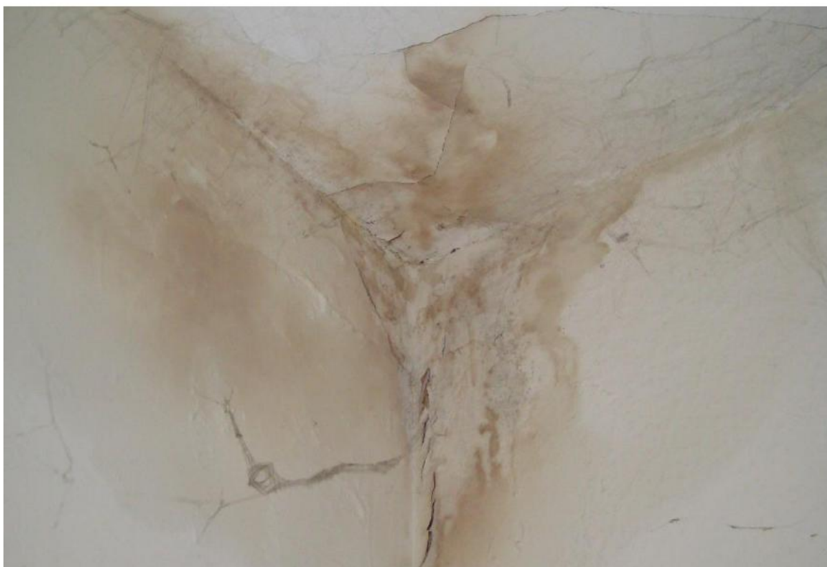
Damp penetration from leaking shower
