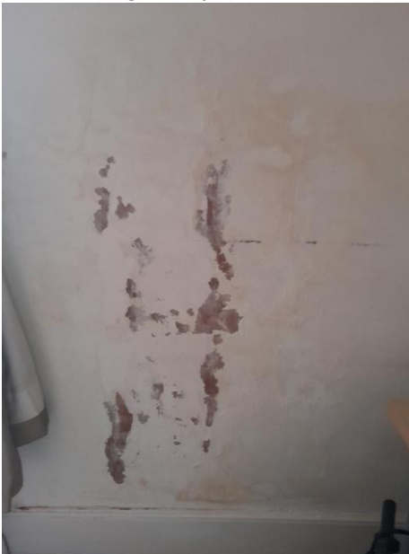
Penetrating damp from defective guttering
