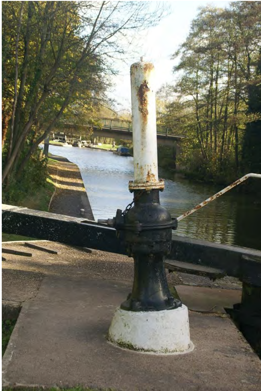
PADDLE GEAR PARTICULAR TO THE BROAD SLUICES
