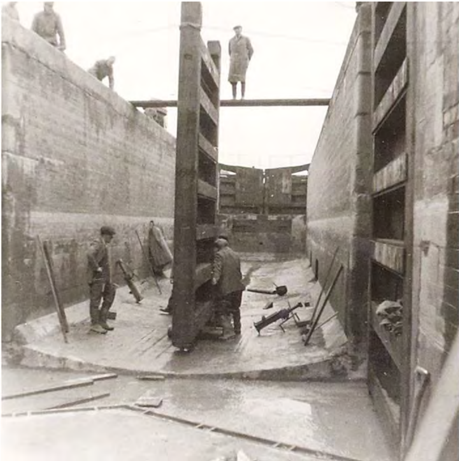
NEW LOCKGATE BEING FITTED IN BROAD LOCK 1958
