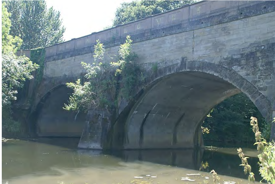
MASONRY ARCH AQUEDUCT WAS CONSTRUCTED FROM SAME STONE QUARRIED AND FLOATED DOWN RIVER IN THE 1790's, THE SAME DECADE AS EARL'S AVON ROAD BRIDGE
