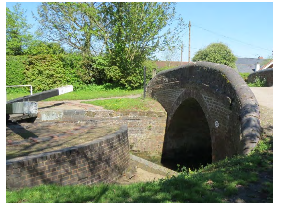
The turnover bridge, 30, has a footpath off to the South west that skirts the village cricket ground. The elegant bridge curves on plan as well as elevation. It appears to have had a concrete saddle to reinforce the deck. The copings sweep up to smooth the passage of the tow ropes over the saddleback copings as the towpath changes sides.
