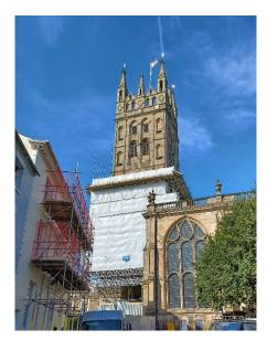
It is a busy junction for pedestrians and vehicles alike; consequently, our immediate priority was to protect the public from falling masonry by erecting netted scaffolding to around half the height of the tower. To do this, it was necessary to implement a comprehensive and costly traffic management programme for the duration of the scaffold build. Under this programme, all three roads were temporarily closed to through traffic.
