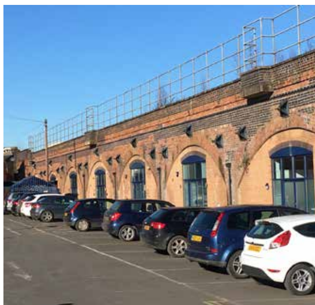
Council leased arches accessed or Court Street Car park
