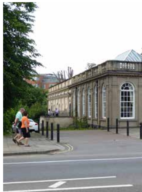
Service Road obstructs route to boardwalk and river
