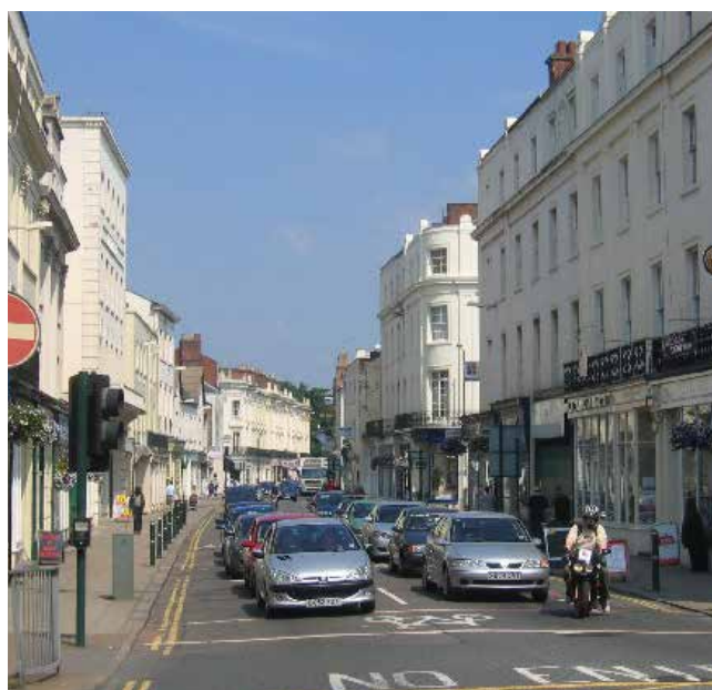
Bath Street is a primary vehicle route from the north of the town.
