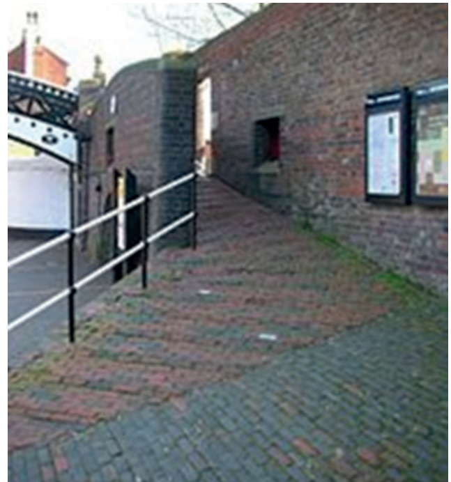
Improved access at Gas Street Basin (Wikipedia)
