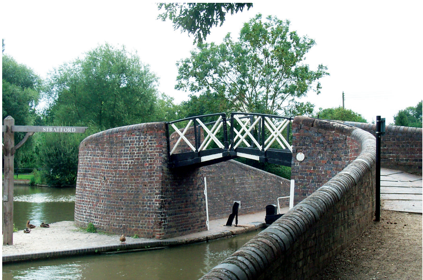
Split Bridge 2m North of Lock 21
