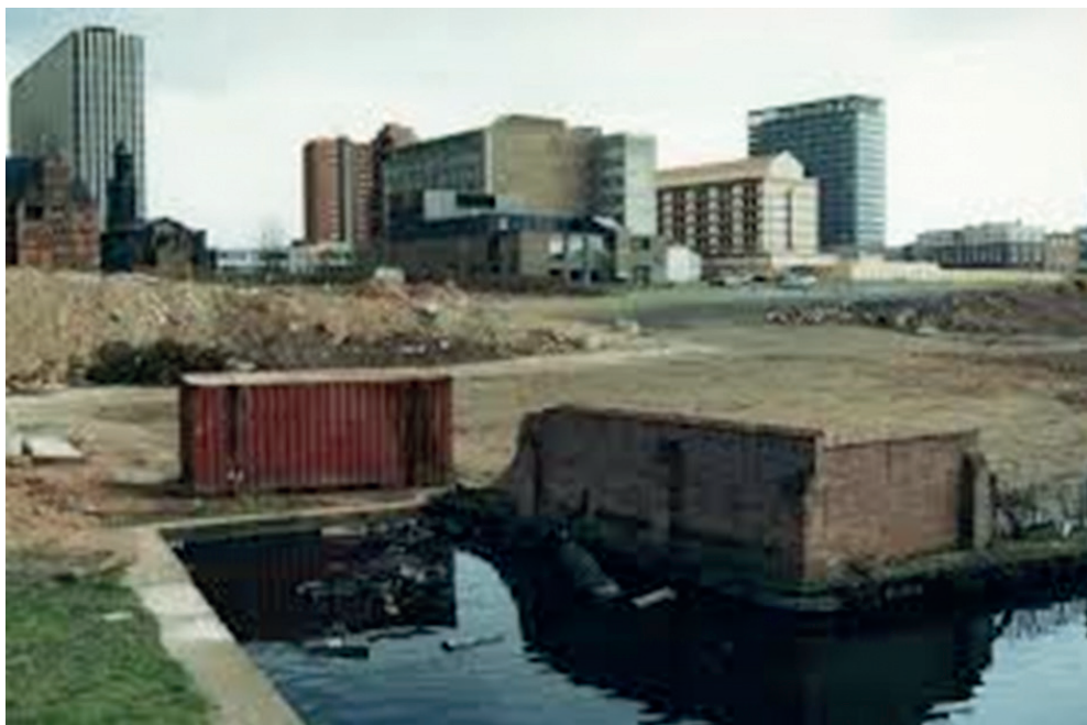
Brindley Place before work was carried out (Urban Buildings)
